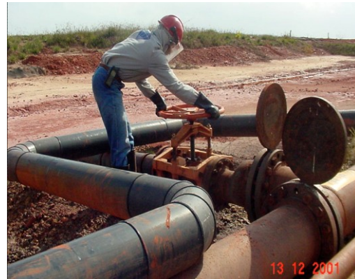
Pictures 4&5: View of the pinch valves and of the HDPE piping installed to operate Upstream
