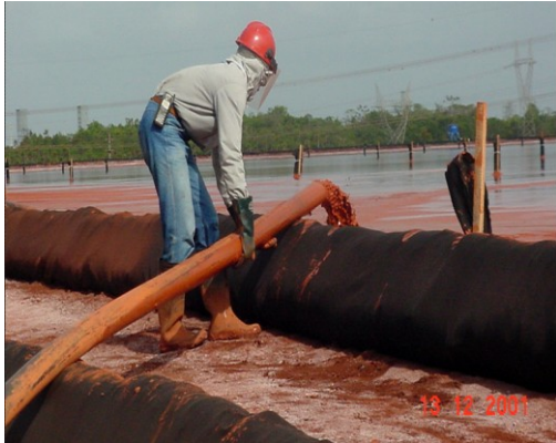
Pictures 4&5: View of the pinch valves and of the HDPE piping installed to operate Upstream
