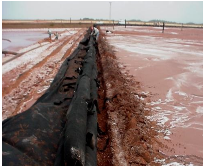
Picture 3- View of the geotextile bags filled with plastic residue forming the low height successive dike
