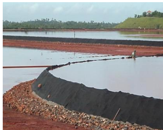
Pictures 1&2: View of the first perimeter dam constructed on RSA 2 surface with refractory bricks (another residue from the plant)
