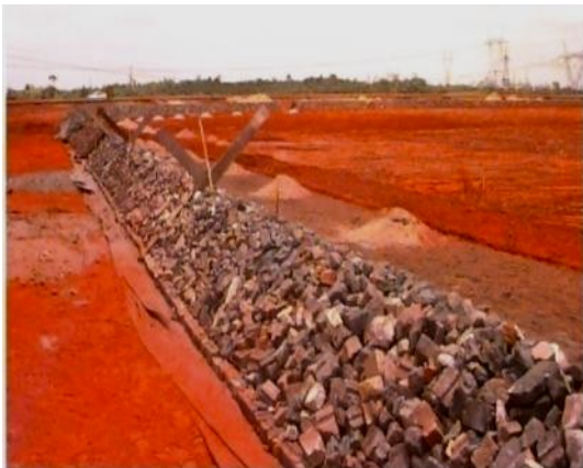
Pictures 1&2: View of the first perimeter dam constructed on RSA 2 surface with refractory bricks (another residue from the plant)
